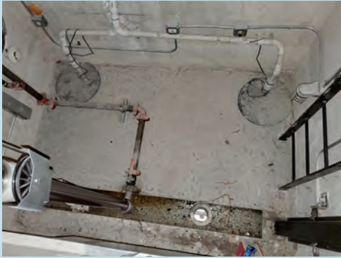
Construction dust from an elevator's installation 15 years prior
