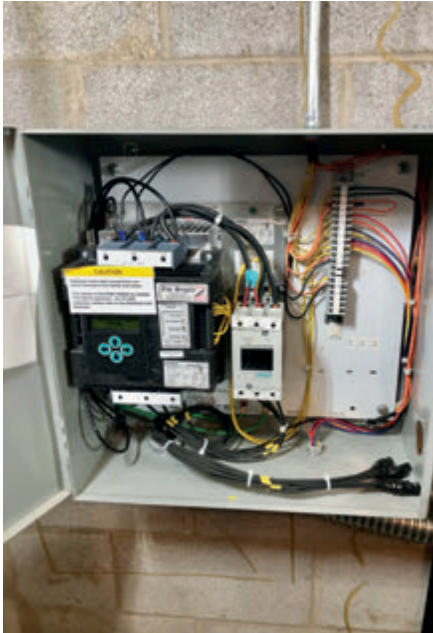
▲ Soft starter with LED fault code display
