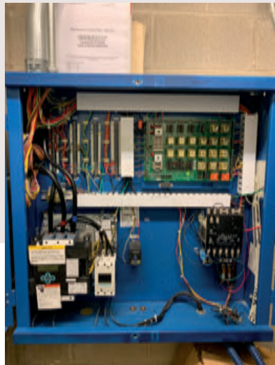
▲ Soft starter after upgrading
